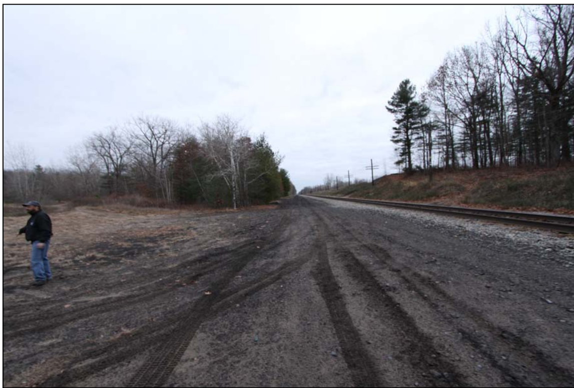
Figure 38. Railroad tracks in Woodlawn Preserve looking south. Originally there were as many as four tracks along this route. A new second high-speed rail has been approved. A wildlife migratory tunnel should be built here at this location. Photo by Don Rittner.
