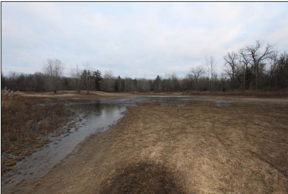
Figure 46. Area east of the pond (on left) flooding the open area. Tree line on the right has been killed from periodic flooding. The levee/berm will be placed along this route to the left to prevent future flooding and this area will be revegetated with native Pine Bush flora. Photo by Don Rittner.
