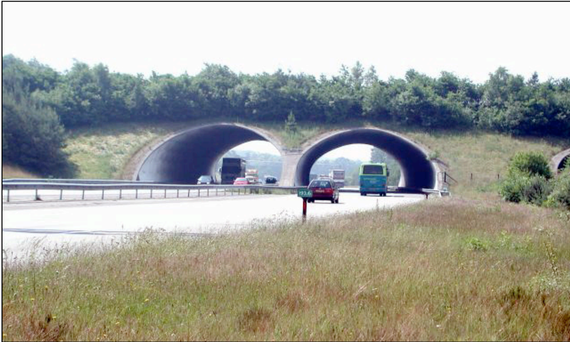
Figure 36. The Cerviduct is one of more than 600 wildlife crossings in the Netherlands. From Wikipedia.
