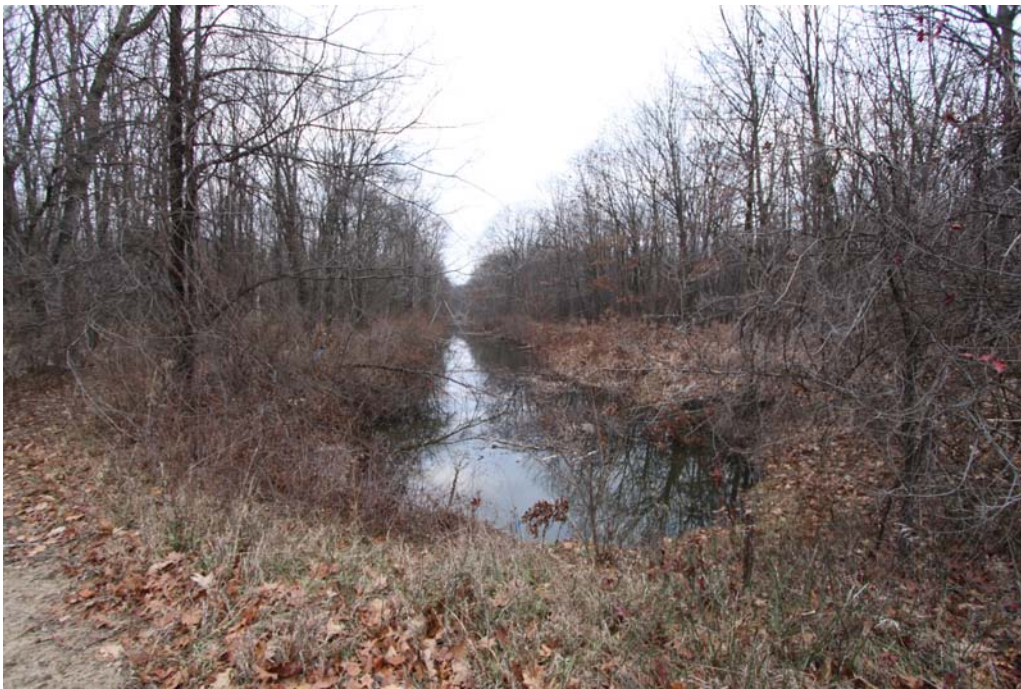
Figure 43. Man made canal drains the lake into the Lisha Kill. Clogging may be increasing the chances of spillover in the preserve. DEC requires maintenance of this canal. See Figure 66. Photo by Don Rittner
