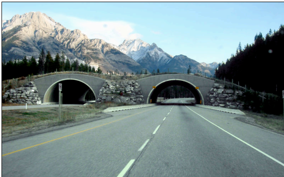
Figure 37. Baniff National Park wildlife overpass. From Wikipedia ( http://en.wikipedia.org/wiki/Banff_National_Park ).
